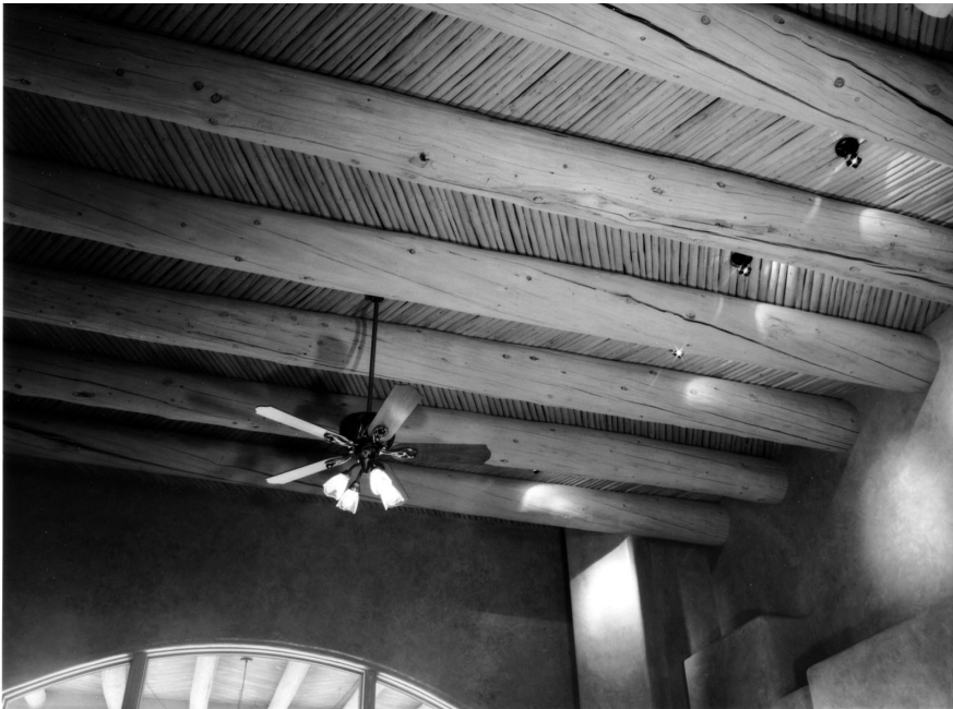
Figure 1. — Viga latilla ceiling. Vigas are the larger diameter poles and latillas are the smaller diameter poles.
